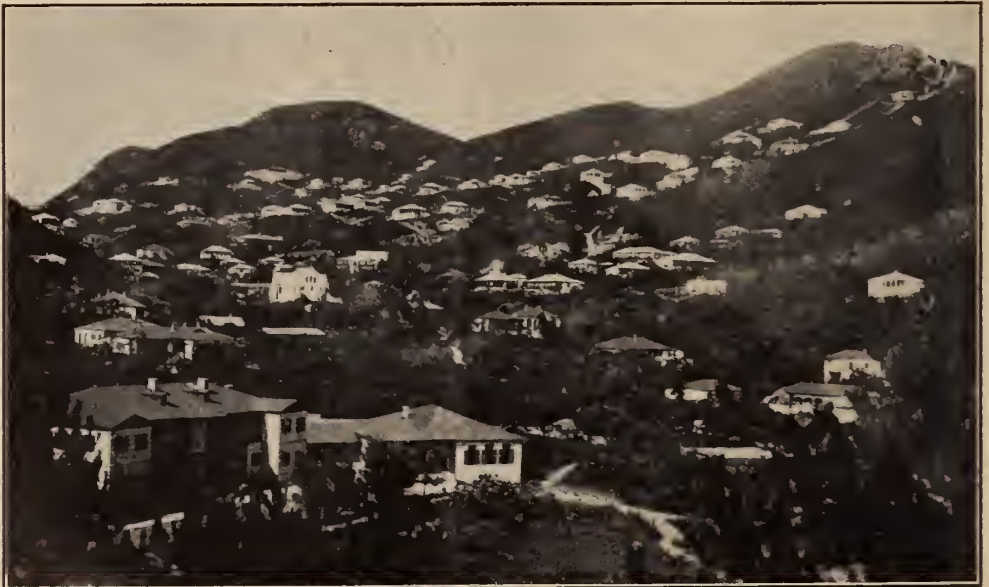
THE VALLEY, WHOSE SLOPES ARE BUILT UP WITH LITTLE STONE BUNGALOWS.
